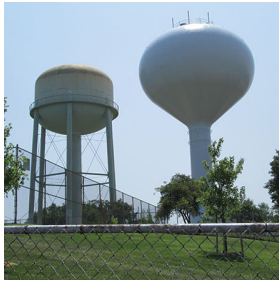
Elevated Storage Tank
